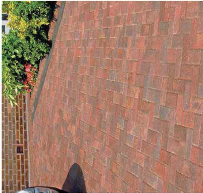
Block Paving and Edging
